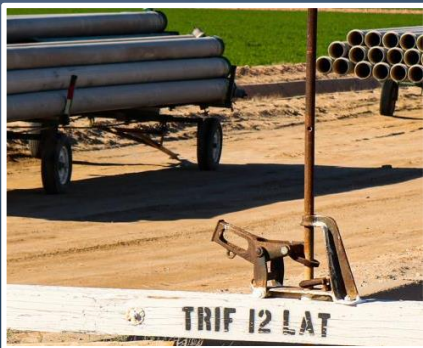
IID-SDCWA Conservation and AAC Lining Transfer/Exchange
