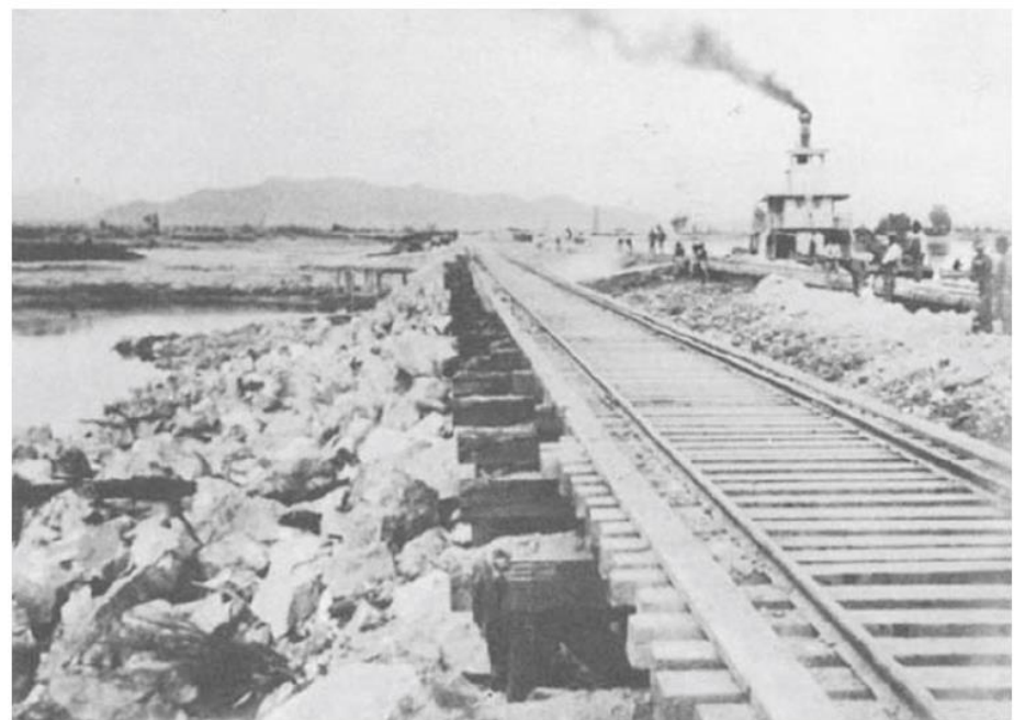
Final repair completed February 1907
