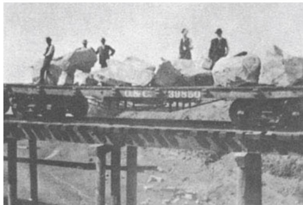
Dumping Boulders to close the breach 1907
