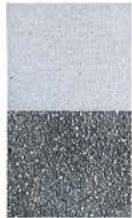
TERRAZZO FLOOR (E) FL-1: EXISTING TERRAZZO FLOOR BY LANDLORD
